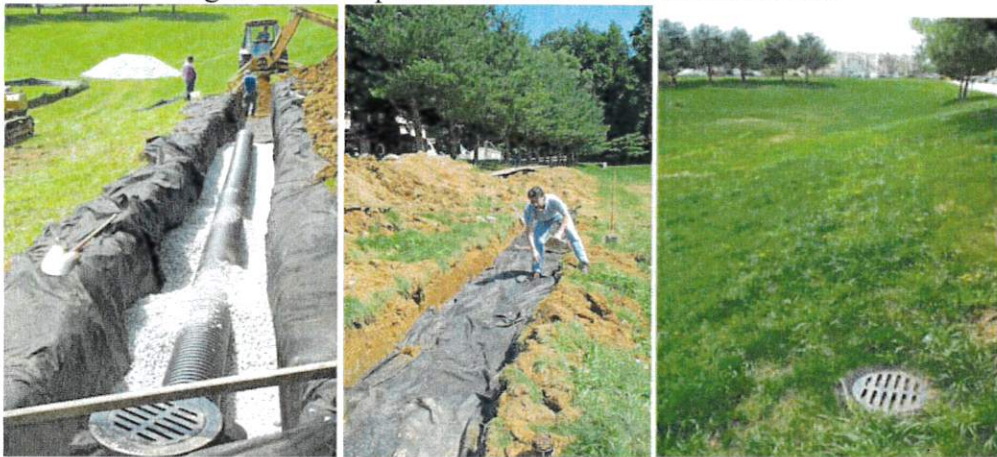
Figure 3: Example of Infiltration Trench Installation
